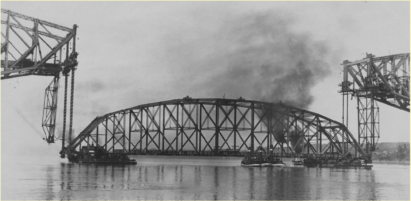
A small fleet of tugs was used to hold the central span in position on September 17, 1917 as the lifting links were being pinned to the span. Library and Archives Canada e011193064
