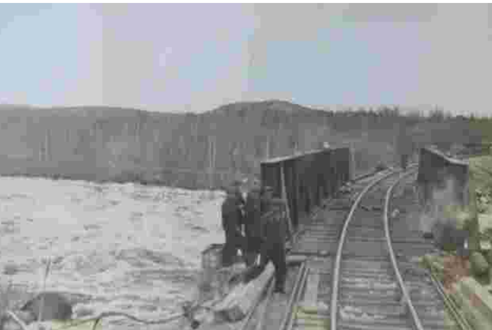
Photo 131: Rattling Brook bridge replacement looking west, MP 256.
