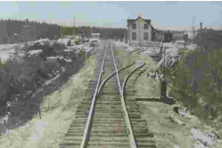
Photo 12: Robinson's Station, MP 480. Gare de Robinson's, PM 480
