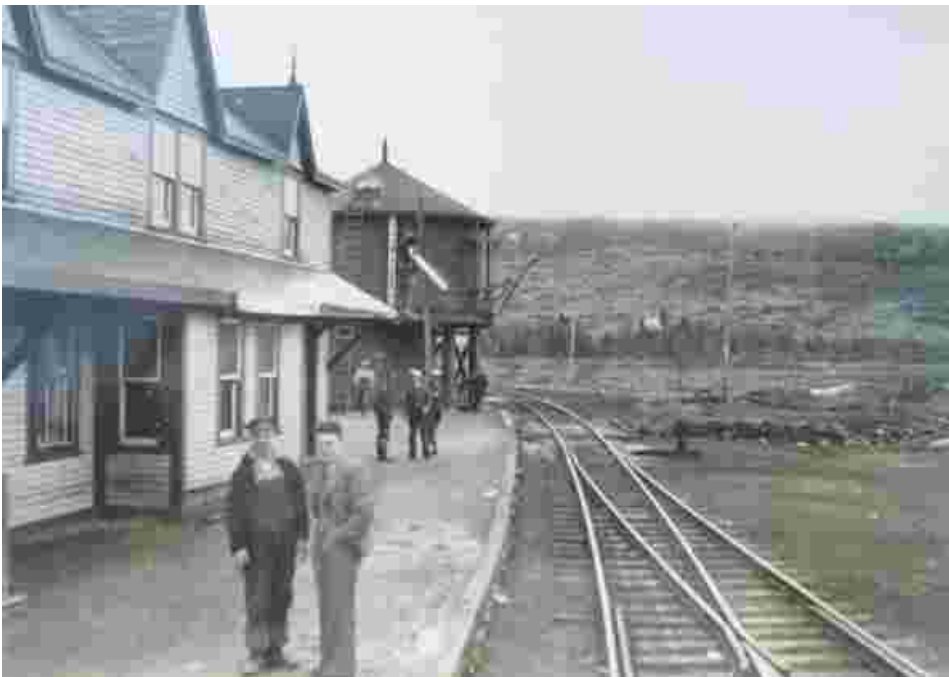
Photo 76: Brigus Junction, station and water tank MP42.
