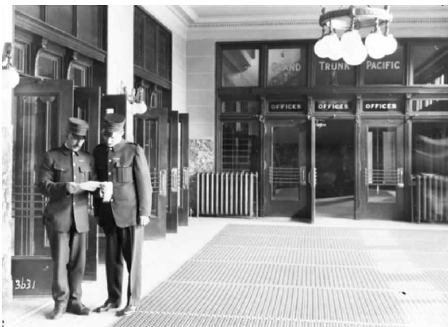
The GTP head offices were located at one end of Winnipeg Union Station and the NTR/CGR at the other. Library and Archives Canada
