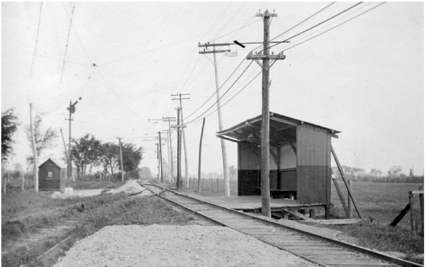
Early view looking north at Blue Bonnets, fresh gravel has been spread between the loading ramp siding and the single track Cartierville streetcar line. Note the switch in the distance curving left into the loop. The track arrangement is protected by a semaphore signal with a signalman's shelter. STM Archives
