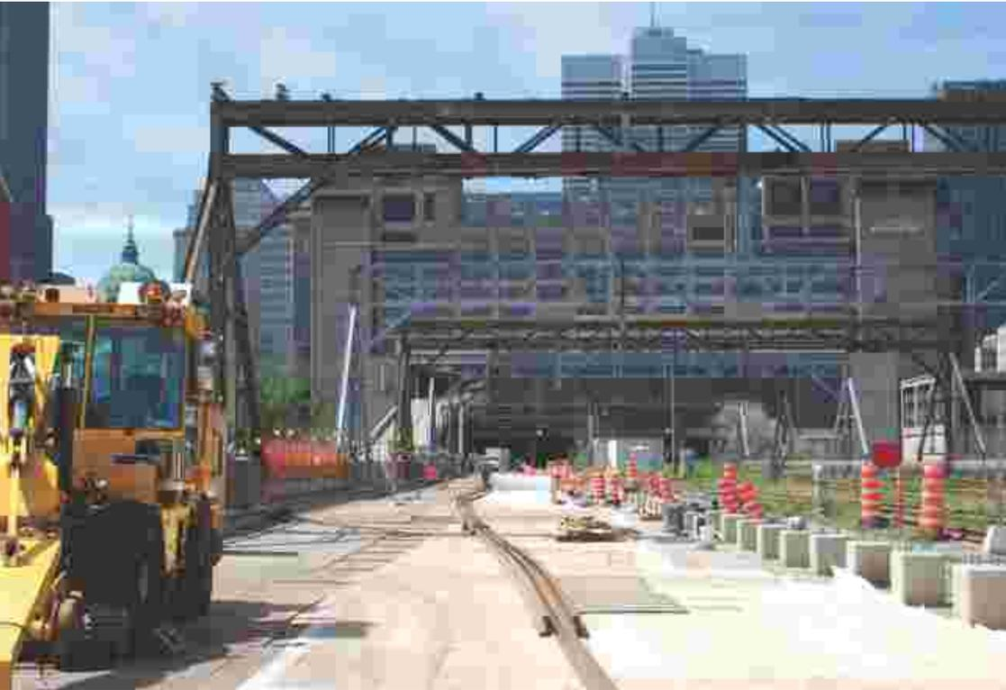
By August 2021 preparations were well underway for the REM entry to Central Station from the south, using the west side of the long established 'viaduct' that carries VIA Rail and exo Saint-Hilaire trains over a number of city streets south of Central Station. Still in place were the steel gantries used for the overhead of the former exo electrified heavy rail operations. REM
