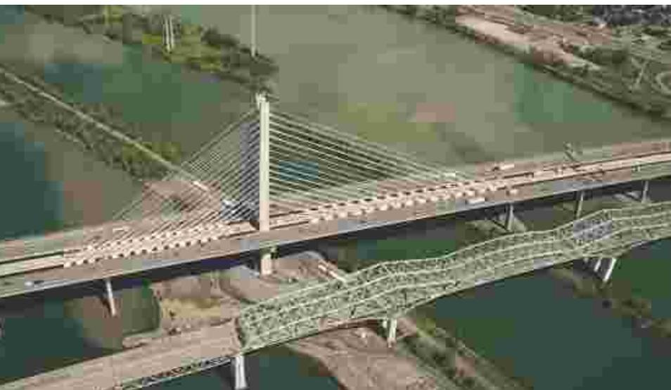
An August 2020 view of the main pylon and cable stays section of the new Samuel-De Champlain bridge, opened in 2019. Clearly visible between the two highway platforms, and separated from them, is the platform upon which the REM will operate. In the foreground is the old Champlain bridge, currently being dismantled. The Saint Lawrence Seaway channel runs from the upper left to the lower right. REM
