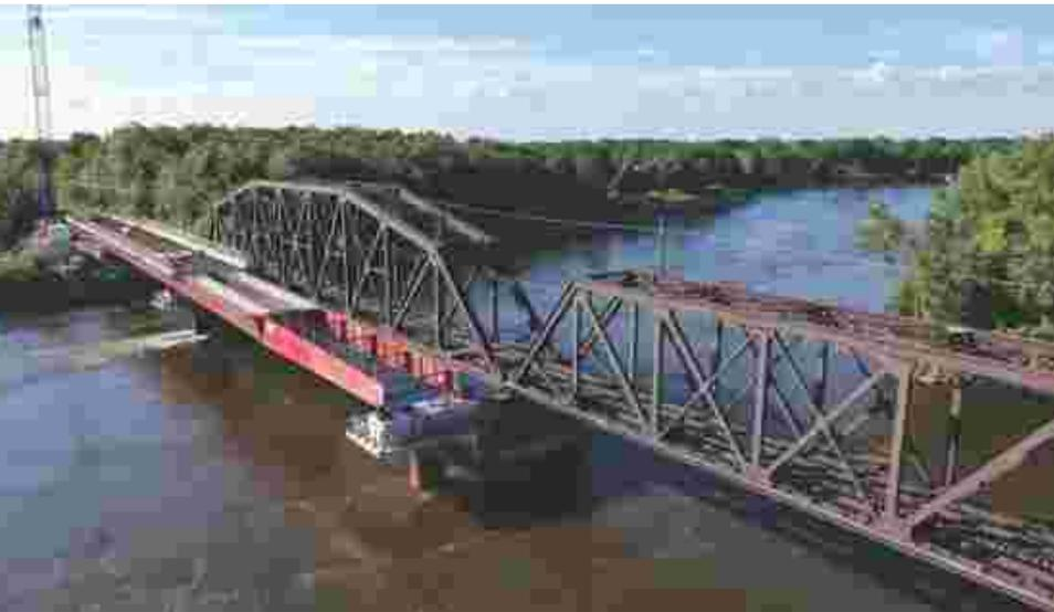
An August 2020 view of the bridges over the larger of the two crossings of the Rivière-des-Prairies, showing construction of the new double track structure. The new spans are being constructed using the 'counterweight launching method.' REM
