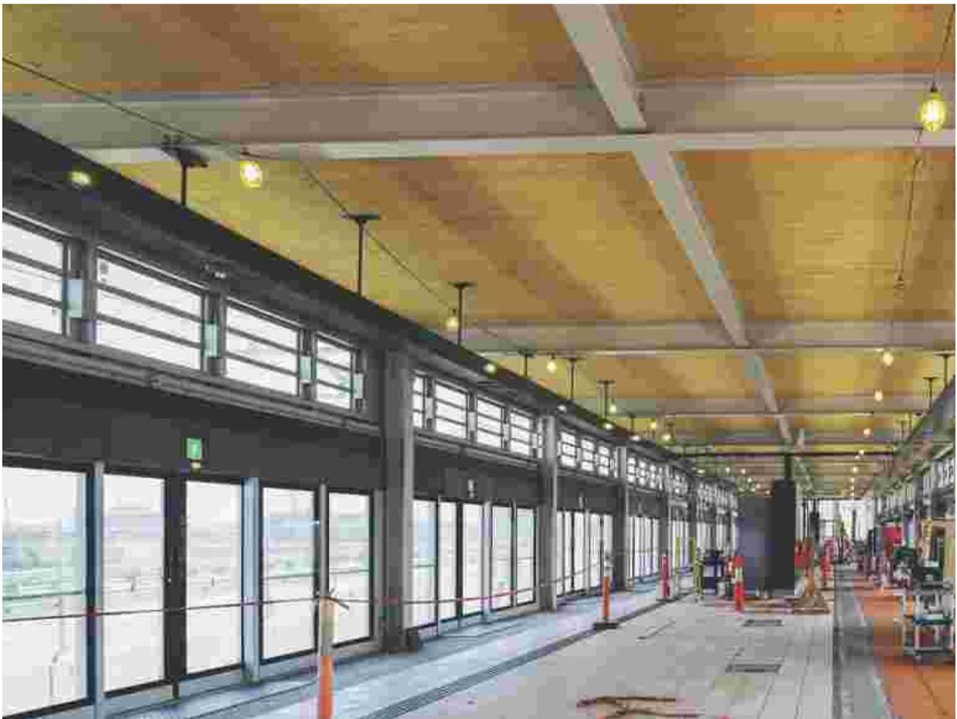
An August 2020 view of the interior of the platform area at Panama station showing platform screen doors and the use of wood as a design component of the interior finish. REM
