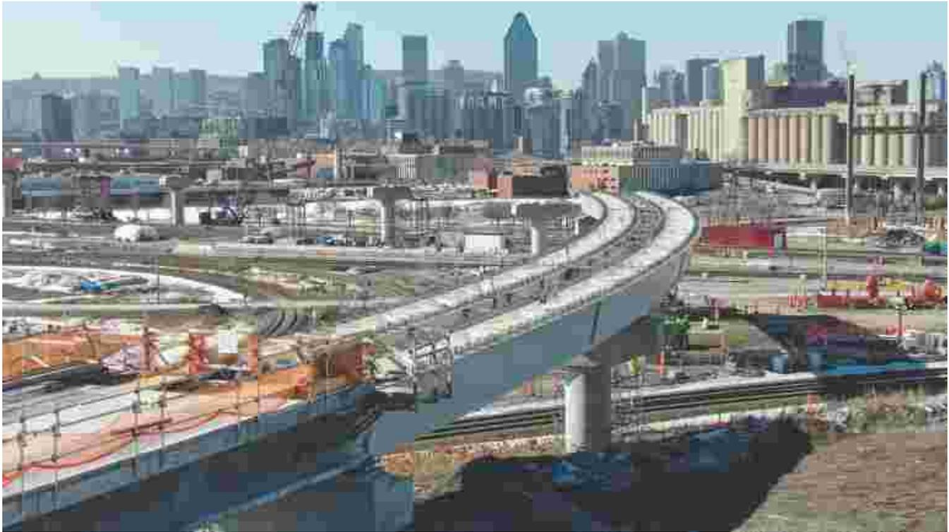
In a March 2021 view with the city's downtown core in the distance, the REM platform enters Pointe-Saint-Charles on massive curved pre-fabricated steel beams, en-route from the Samuel-De Champlain bridge to Central Station. To the right of the photo the rail lines lead to the Victoria Bridge; to the left, they lead to Gare Centrale, the VIA coach yard and maintenance facility, to CN's Pointe-Saint-Charles yard and to the CN Kingston subdivision. REM
