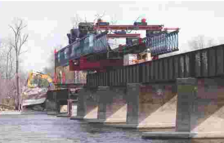
In April 2021 a gantry works at the beginning of the project to replace the single track bridge over the Rivière-des-Mille-Îles with a new double track structure. Each old span was lifted and moved to enable the height of its old piers to be reduced, then replaced. By this process a platform was created upon which the work to create the new span and piers could proceed. Ian MacDonald
