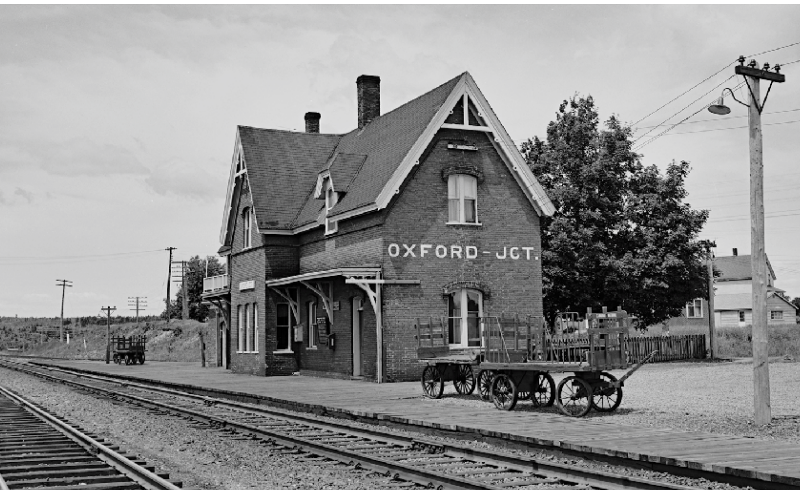
Oxford Junction Station. Harold Jenkins | La gare de Oxford Junction. Harold Jenkins
