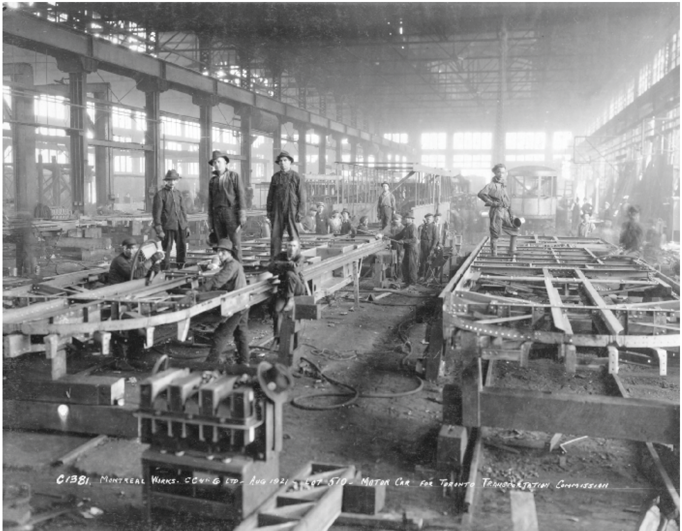
From wood to steel. Interior view of Canadian Car & Foundry Limited in Ville St. Pierre, Quebec. Under construction are the 2300 series Peter Witt streetcars for the newly formed Toronto Transportation Commission in 1921. CRHA / ACHF Exporail Archives, Fonds Canadian Car & Foundry
