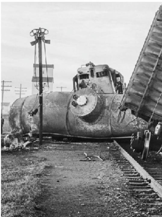
This tank car full of gasoline derailed and split open following the crash between two trains at Carbondale station. The fuel ignited, incinerating the station and three people in it. Provincial Archives of Alberta
