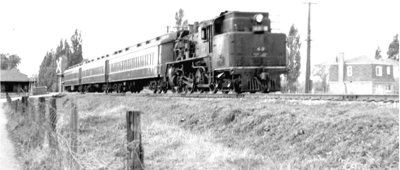
The GTR / CNR X-10-a 4-6-4T's operated in a bidirectional fashion. Westward to Dorval and Vaudreuil, normal practice was to operate smokestack / boiler first. Eastward to Montreal, they normally ran coal bunker first such as No 49 is seen doing here leaving Dixie station for Montreal with an all steel commuter consist circa 1954. Leonard A Seton, Smail collection
