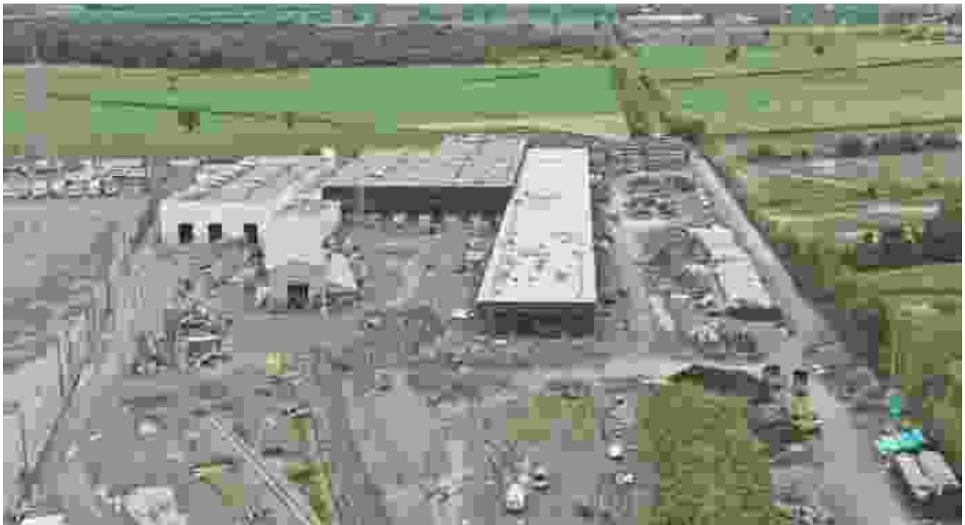
Aerial view of the Saint-Eustache Maintenance and Service Centre, August 2022. REM
