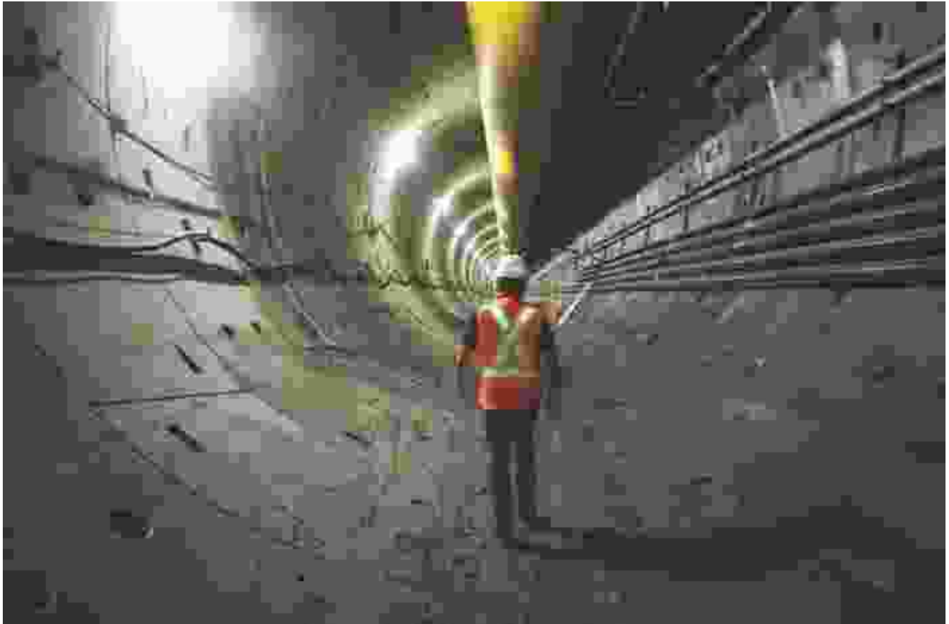
Interior view of the airport tunnel, ready for the installation of railway infrastructure. REM
