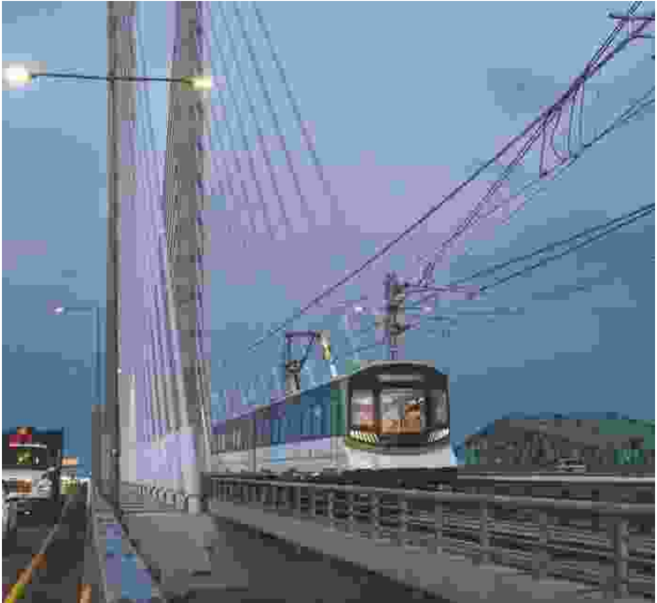
First run over the new Samuel-De-Champlain bridge and on to Central Station on July 27, 2022. Thierry DuBois, REM
