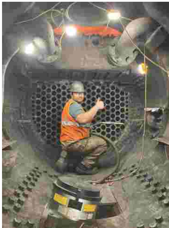
Dean Pratt works inside 2816's boiler as tubes are removed for the 15-year inspection.
