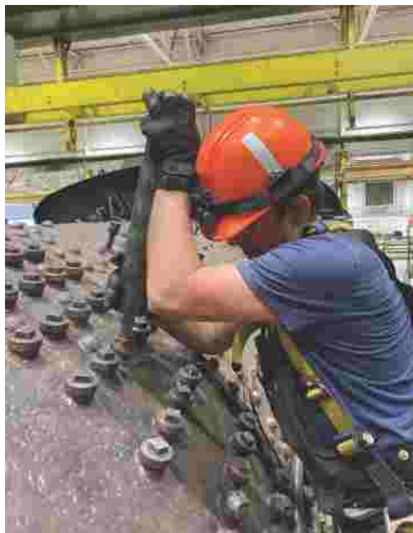
Krys Bialorucky assists with stay bolt work on 2816's firebox.
