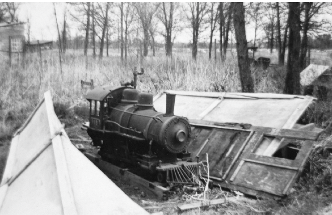
Lying amongst the debris following the demolition of the amusements at River Park was the miniature locomotive. There is no information as to its fate. Archives of Manitoba P1250
