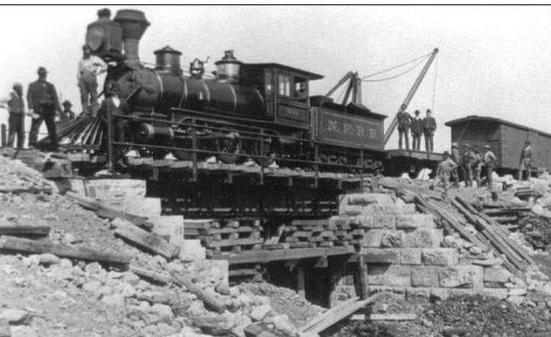
This bridge reconstruction operation, believed to date from the early 1890's, was photographed along the shoreline of Conception Bay, about 20 miles west of St. John's, on the route of the original railway line to Harbour Grace. AR Penney collection
