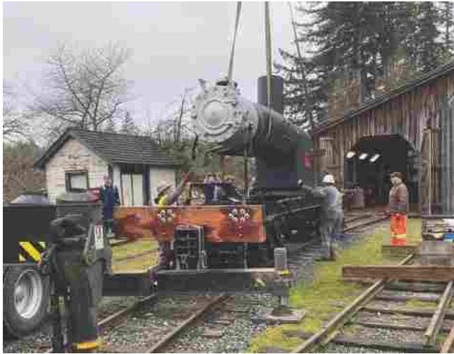
Boiler lift, February 2, 2022
