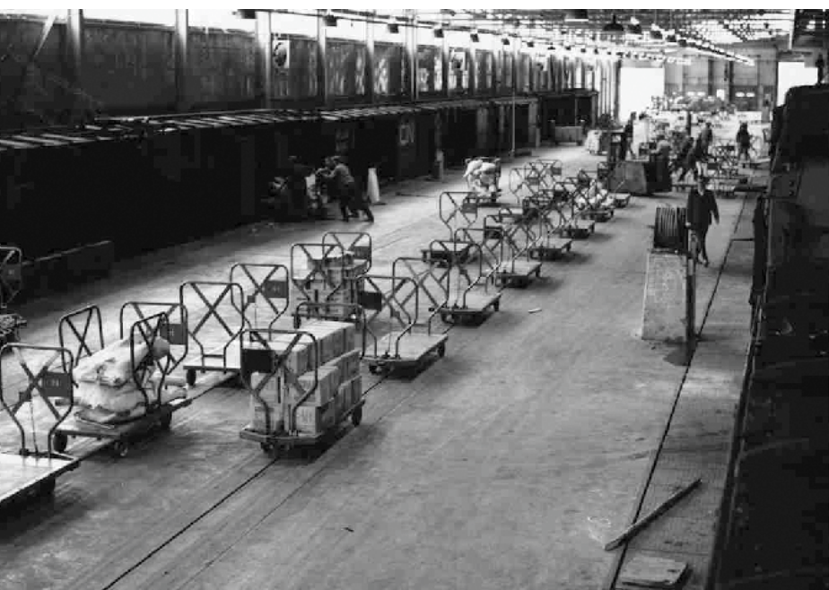
The transfer shed at Port aux Basques, circa 1968. Although still quite labour intensive, the transporting of mainland freight cars across the gulf significantly reduced handling and delays to cargo. The Newfoundland cars are on the narrow gauge track at left, and the mainland ones on the right. Marine Atlantic archives
